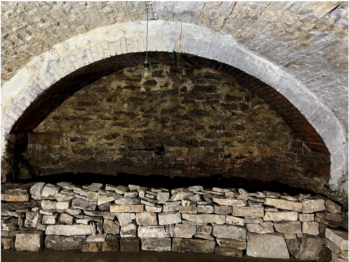
Brick arch at end of boiler room.
